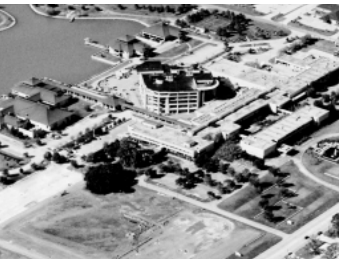
Aerial photo of the Pennington Biomedical Research Center campus with construction of the Basic Science Laboratory Building underway
