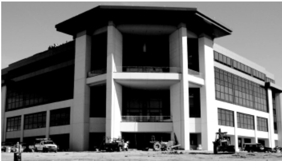
Construction in process on the Basic Science Laboratory Building
